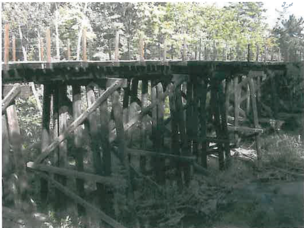
Figure 4: View of trestle substructure over Los Gatos Creek
