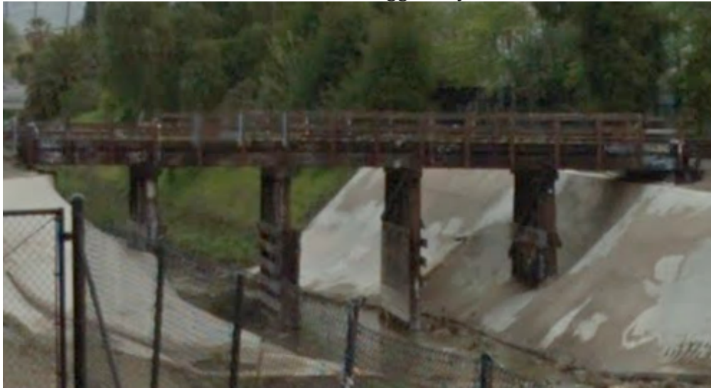
3. Western Pacific over Silver Creek at Eggo Way. Demolition Planned. 22
