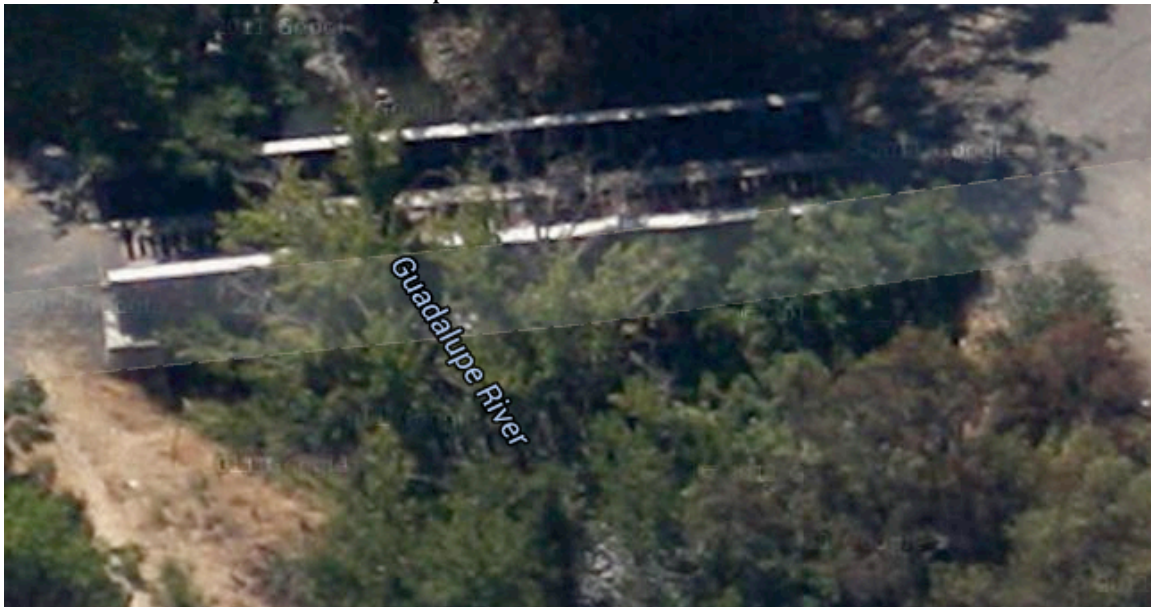
4. Western Pacific over Guadalupe River at Falcon Place. Demolition Planned. 23
