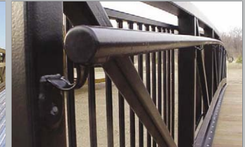
Vertical Picket/Pipe Handrail
