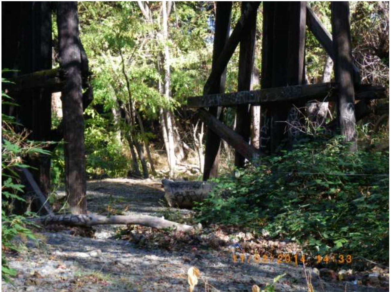
Photo #13. Large wood collected on railroad trestle pier within bankfull channel. 3 November 2014
