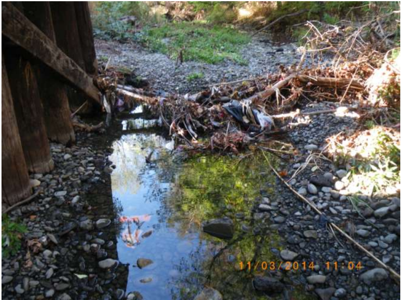
Photo #12. Shallow pool under railroad trestle. 3 November 2014
