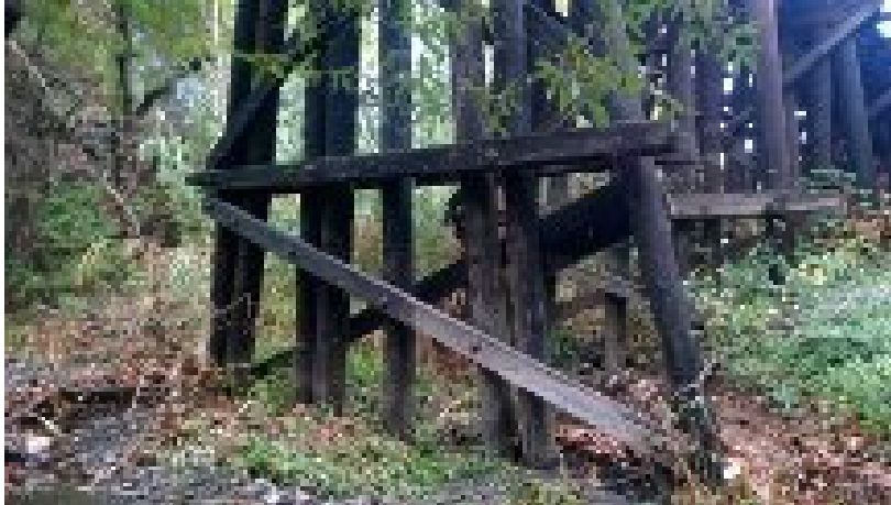
Pile bents showing doubled piles, from Los Gatos Creek bed
