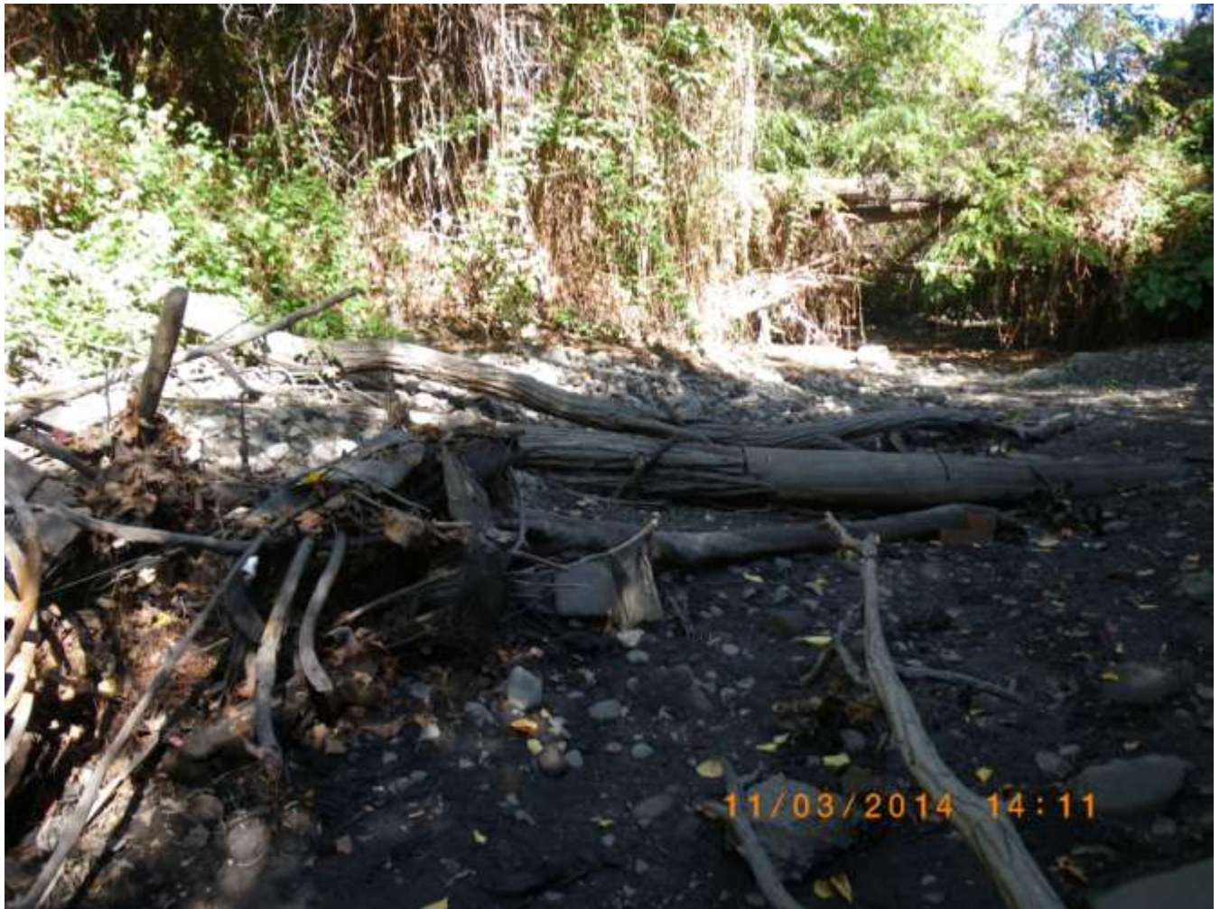
Photo #5. Large woody debris in dry low-flow channel (evidence of cutting) upstream of the railroad trestle. 3 November 2014
