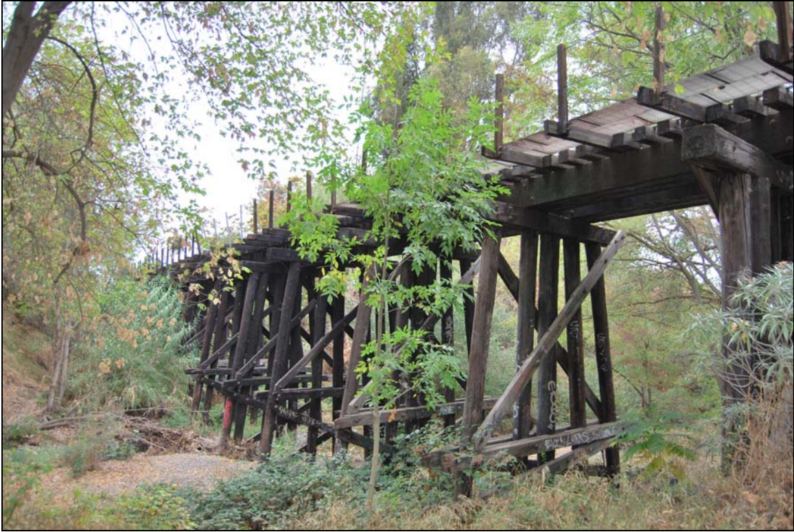
Figure 6: Trestle understructure, view to the north
