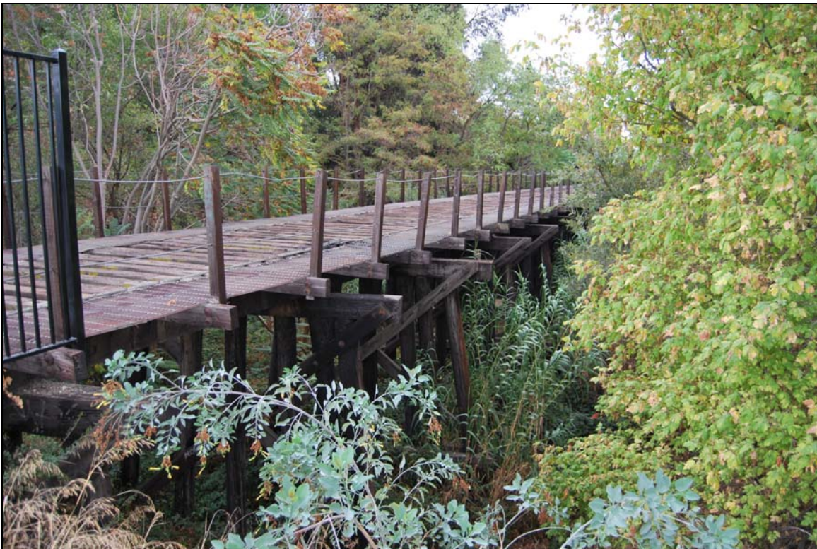
Figure 5: View southeast along trestle
