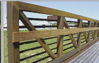
Safety Rail/Wood Rub Rail
